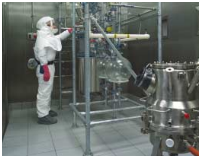
Degussa's Raylo facility in Edmonton, Alberta, Canada.
